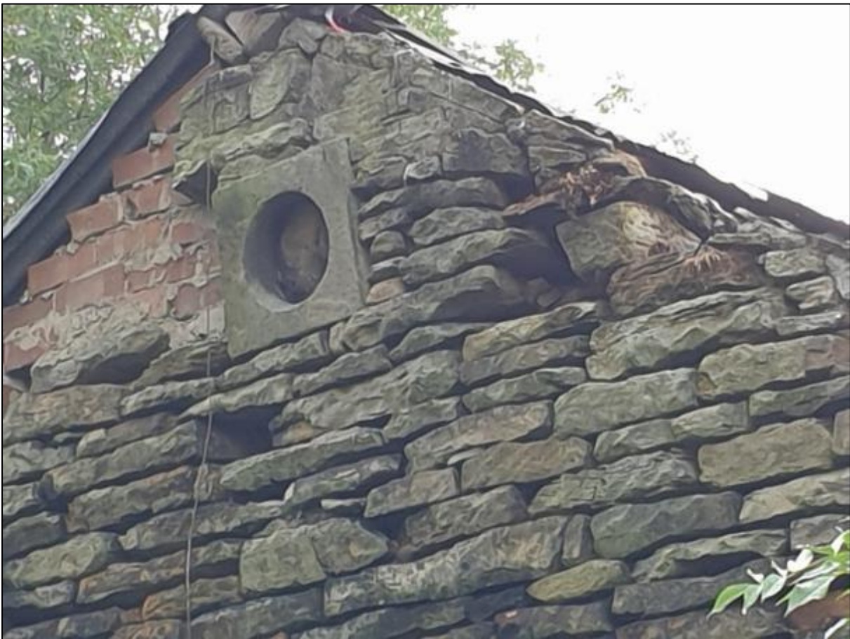
Plate 9 Close up of owl hole within the western elevation of the northern outbuilding
