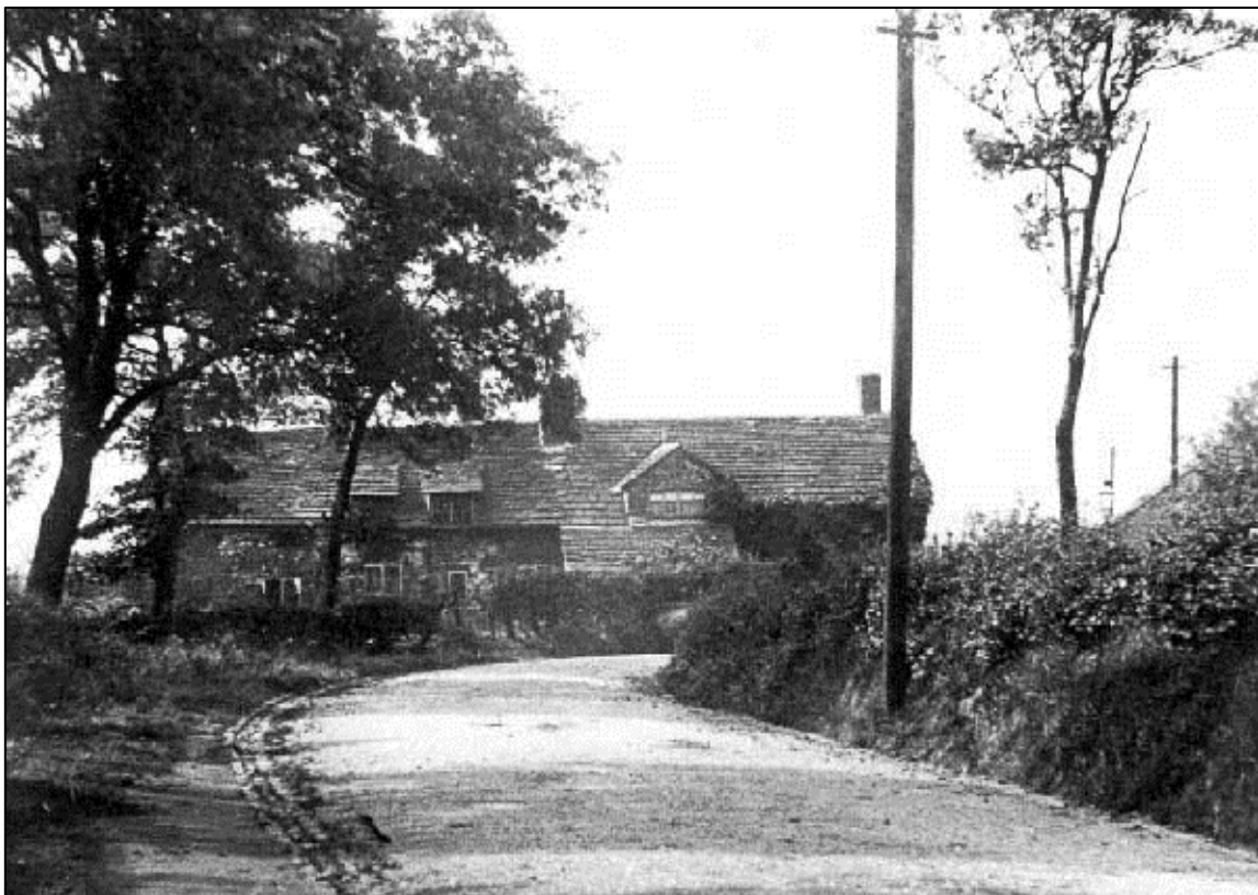
Plate 12 19 th century photograph showing the view of Apethorn farmhouse from Apethorn Lane to the east. This aspect is currently obscured to a certain extent by the overgrown roadside hedge
