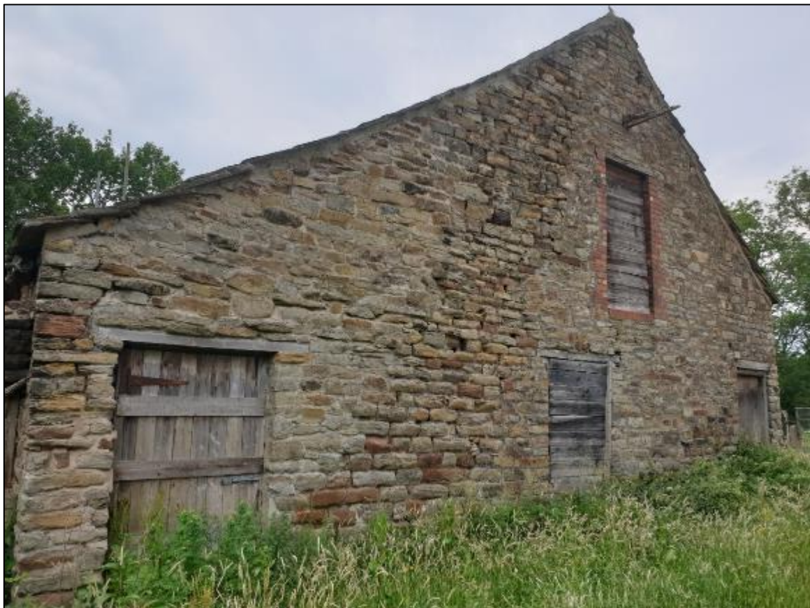
Plate 8 Eastern elevation of the combination barn shows the entrances for the cows as well as a later taking-in door
